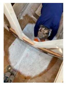
12. the first GRP being applied to the inner skin. This ended up being four layers of CSM and biax with increasingly large overlaps, all using vinylester resin.
